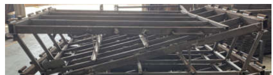
Ramps no mesh on yet
